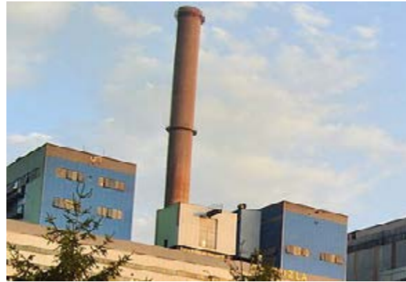
Thermal Power Plant in Tuzla Photo: Wikimedia Commons/Edinwiki
